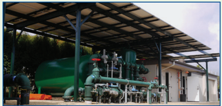
Filter media was replaced at San Ricardo Well
