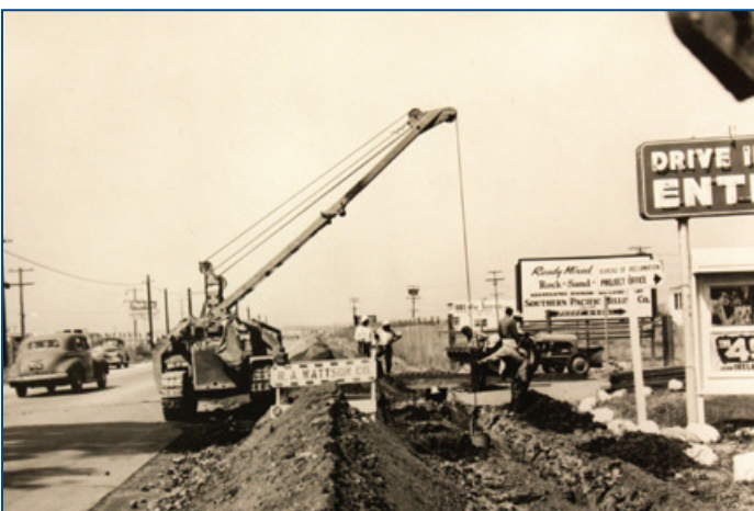
Goleta Water District infrastructure being installed in the early 1950s.
